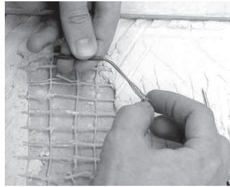
**Step 3.6.** Loosen the braid by pushing back on the braid about 1/2" and cause the ends of the heating wires to be exposed.
