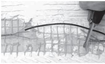
**Step 4.12.** Cut the jumper wires shorter, if necessary, so that they overlap the stripped ends of the heating wires.
