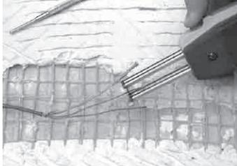
**Step 4.10.** Use the thermal wire strippers to carefully strip off exactly 1/2" of the insulation from the heating wires. Count the little heating elements to make sure none were cut off and thereby cause a hot spot or possible failure. A fiber strand may also be found among the heating elements. There is no need to separate or remove this fiber strand.
