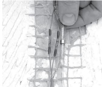
**Step 3.16.** Slide a ground solder tube onto the longer ground wire. Overlap the ground wires and twist them to help hold them together. Slide the ground solder tube over the twisted ground connection centering the connection under the ring of solder.
