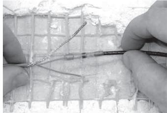
**Step 4.15.** Place the heating elements and jumper wire ends alongside each other. **Lightly** twist the elements together to better join them. Slide the solder tube over the twisted elements and over the edge of the insulation on the jumper wire. Make sure the twisted wires are fully inside the solder tube and located between the adhesive bands at the ends of the solder tube. If this is not done correctly, the elements may pull out and cause the splice to fail.
