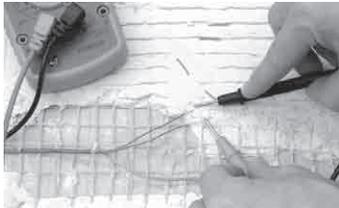
**Step 4.11.** Use the digital multi-meter and TDR at this repair location before proceeding. Check for any additional damage locations in the heating cable by "looking" in both directions. For assistance in using these instruments, consult the instructions that came with them.
