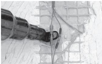
**Step 3.15.** Repeat Steps 3.12 through 3.14 for the other heating wire splice. Make sure to avoid reheating or scorching the first splice while working on the second. It may require a heat shield like a wet cotton rag or a piece of tin to protect the first splice and the insulation of the heating wires.
