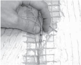
**Step 3.13.** Pull the heating wires together to overlap the heating elements of both leads. Lightly twist the elements together to better join them. Slide the solder tube over the twisted elements, centering the elements between the gray adhesive bands. If this is not done correctly, the elements may pull out and cause the splice to fail.
