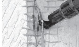
**Step 3.17.** Be sure to avoid reheating or scorching the heating wires or splices, using a heat shield again if needed. Heat the tube to shrink it completely and cause the solder to flow into the twisted ground wires completely. When it cools, the connection should be secure.
