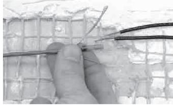
**Step 4.14.** Slide a solder tube over one of the heating wires on one lead of the heating cable, or position it on the jumper lead if that makes joining the wires easier.
