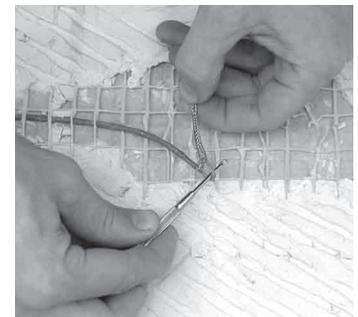
**Step 4.8.** Use the small screwdriver, paper clip, fingernail, or similar instrument to pry between the braid and make an opening through which to pull the heating wires. Pull each wire through the braid.
