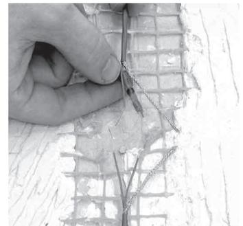
**Step 3.12.** Slide the solder tube over one of the heating wires.
