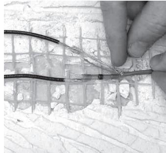
**Step 4.18.** At the other end of the jumper wires, slide a heating element solder tube over a heating wire or its jumper wire, whichever is easier for you to position the tube out of the way and allow for easy access to the ends of the wires. REPEAT Steps 4.14 through 4.17 to complete the heating element jumper wire connections.
