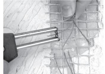
**Step 3.10.** Use the thermal wire strippers to carefully strip off exactly 1/2" of the insulation from the heating wires. Count the little heating elements to make sure none were cut off and thereby cause a hot spot or possible failure. A fiber strand may also be found among the heating elements. There is no need to separate or remove this fiber strand.
