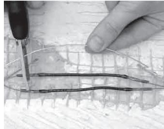
**Step 4.19.** If necessary, cut the ground jumper wire shorter so that it overlaps the ends of the ground wires by about 1/2" to 3/4".
