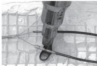
**Step 4.17.** REPEAT Steps 4.14 through 4.16 for the other heating wire. Be sure to avoid reheating or scorching the first heating wire splice, using a heat shield like a wet cotton rag or a piece of tin if needed.
