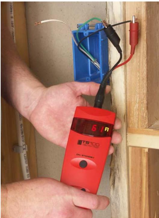
This picture shows the Fault Finder connected to the power leads at the work box on the wall. Black test lead is connected to the cable's green ground lead, red test lead is connected to the black power lead.
