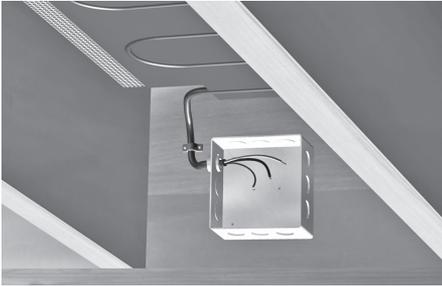
Suspended or unfinished ceilings below the mats allow for installation of junction boxes in the joist bays.
