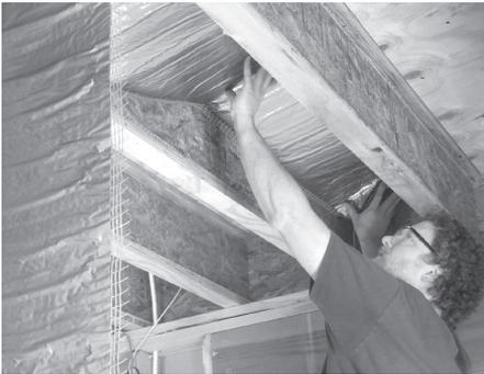
**Test fit the mat between the joists before stapling the mat to the joists.**
