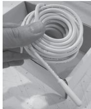
**Floor sensor is included in the SunStat thermostat packaging. This must be installed in the floor with the mat.**
