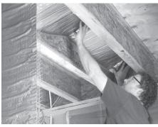
Test fit the mat between the joists before stapling the mat to the joists.
