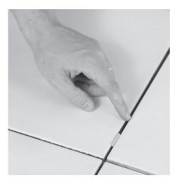
Method 3: Remove the grout 1/4" to 1/2" deep. Install sensor. Reinstall grout over the sensor and sensor wire.
