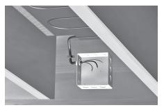
Suspended or unfinished ceilings below the mats allow for installation of junction boxes in the joist bays.
