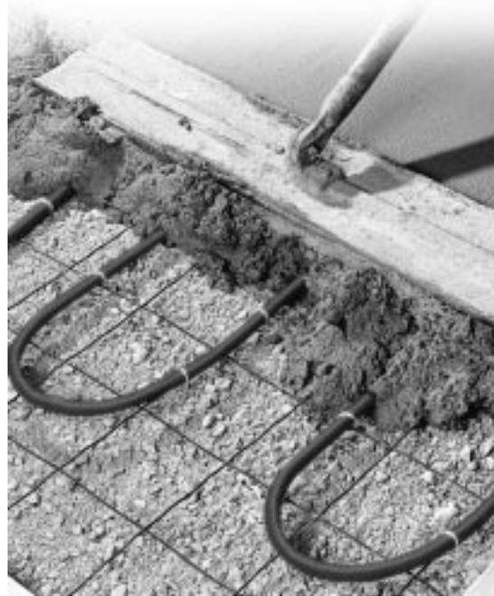
radiant slab faster than a boiler can produce it. Basements and slabs installed in hillsides should have good drainage to carry any subsurface groundwater away from the site. The slab should be placed above an ample amount of crushed rock or gravel.
