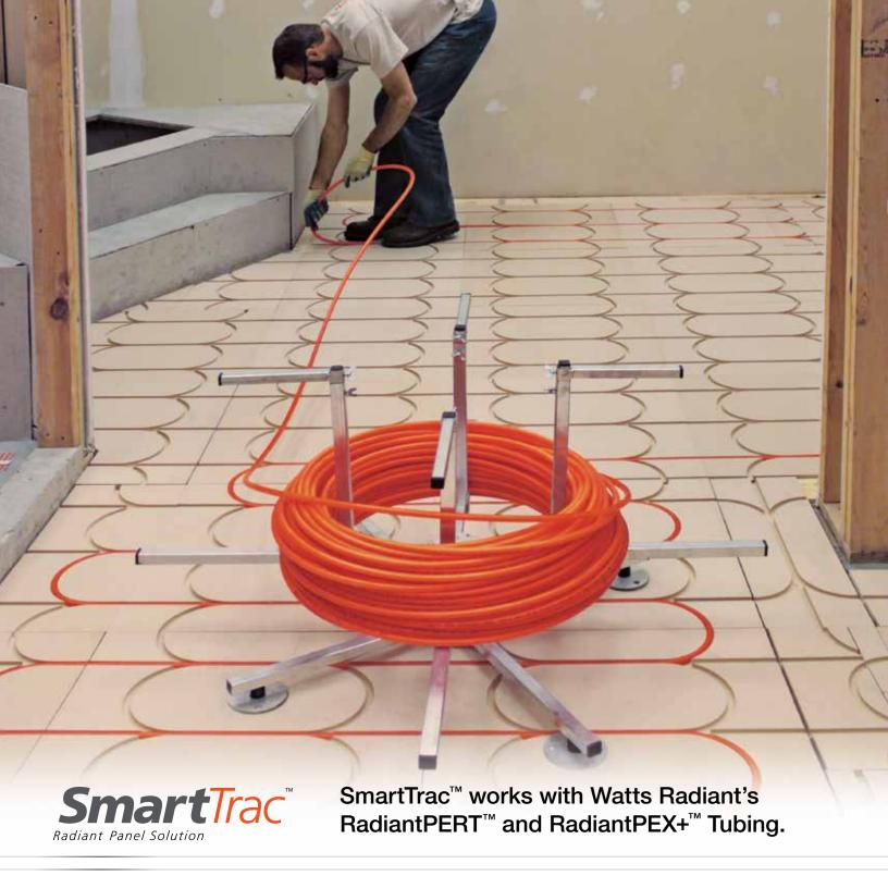
SmartTrac<sup>™</sup> is a non-structural, modular panel system, designed to simplify radiant heating and cooling installations in subfloor, wall and ceiling applications.
