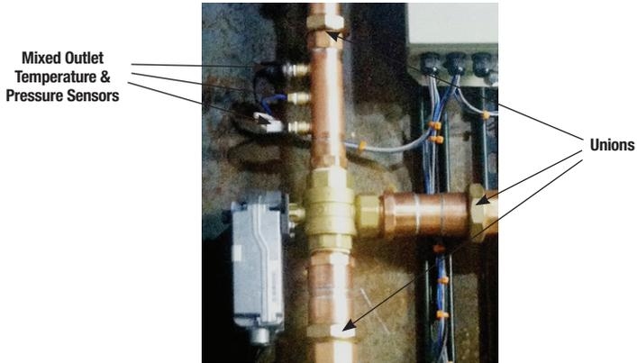
5. If replacing the valve remove the NPT couplers, union fittings, and actuator mounting plate from the old valve and transfer them to the replacement valve for reinstallation.
