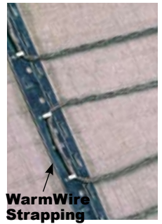
The WarmWire is held in place by WarmWire strapping attached to the subfloor or backerboard.
